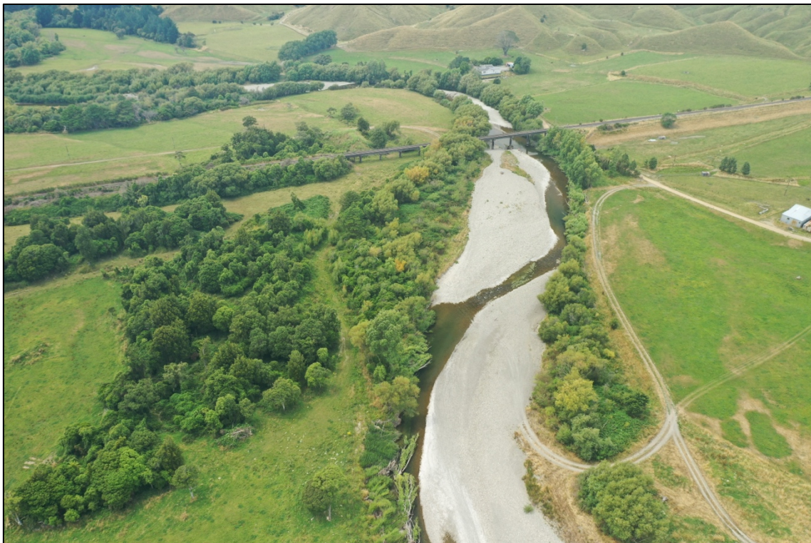
Figure 2: Looking downstream over the Mangatainoka River at Mowbrays Road. Mowbrays Rd can be seen behind the rail bridge on the left of the river.
