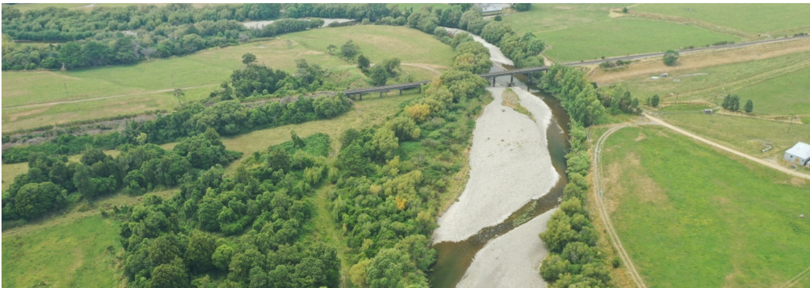
Looking downstream over the Mangatainoka River at Mowbrays Rd. Image: Thomas Kay (Kāhu Environmental).
